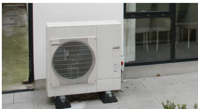
**Figure 2: Air Source Heat Pump Outdoor Unit**
